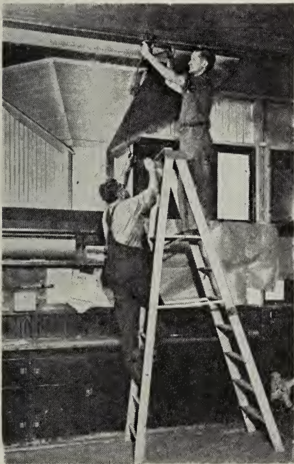
This new heavy duty platform ladder made by the Dayton Safety Ladder Company, is said to be safe for two men to work from.
